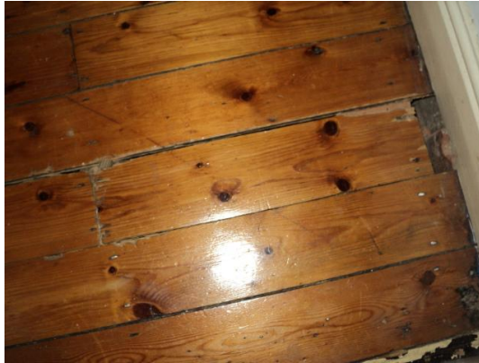
Damaged floorboard
