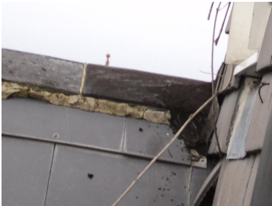
Repair to rear ridge
