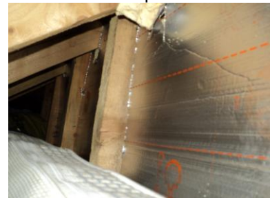
Insulation around loft conversion
