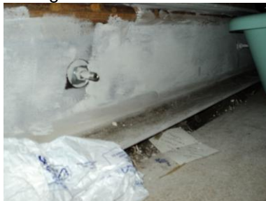
Steel supporting joist to loft
