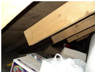
Strengthened rafters to loft
